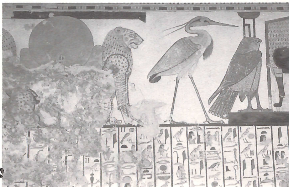
Wall painting of the tomb of Nefertari showing a variety of animals and birds with religious text underneath. To the left is an area that had deteriorated due to salt crystallization behind the plaster layer.
